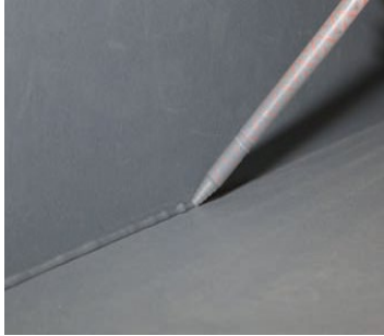
Apply 1/4" bead along seam of base and floor
