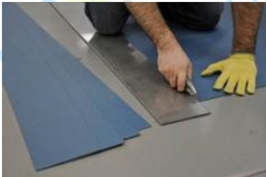
Turning 5' x 8' sheets into 6" x 8' strips
