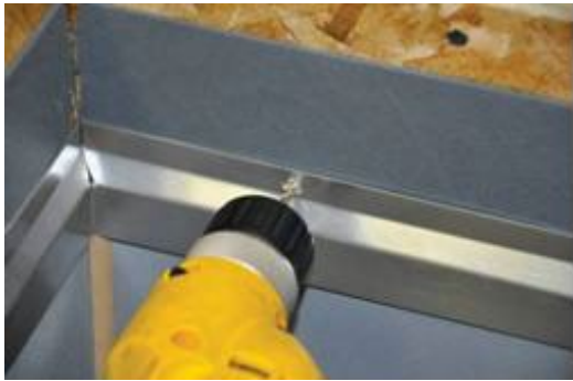
Pre-drill using 1/8" drill bit
