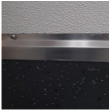
Cove cap on wall
