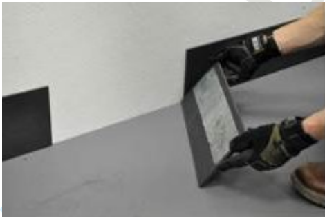
Using web reinforced tape
